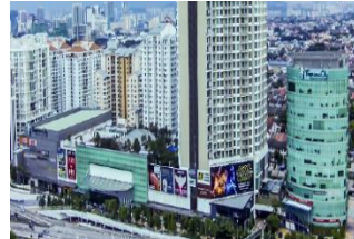
3 Damansara (formerly Tropicana City Mall) & Tropicana City Office Tower, Petaling Jaya
