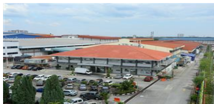
Sunway REIT Industrial – Shah Alam 1
