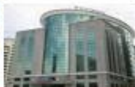
Wisma Technip (a)
