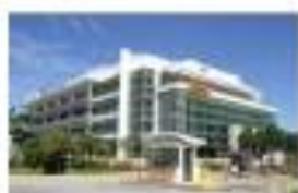
Quill Building 4 - DHL 2 (b)
