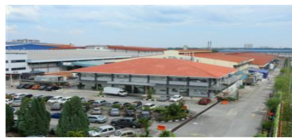
Sunway REIT Industrial – Shah Alam 1
