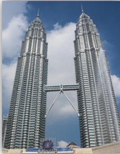
PETRONAS TWIN TOWERS
