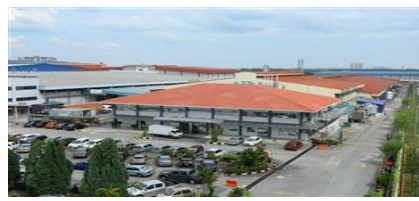
Sunway REIT Industrial – Shah Alam 1
