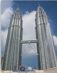
PETRONAS TWIN TOWERS
