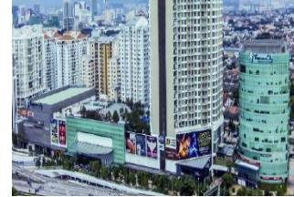
Tropicana City Mall & Tropicana City Office Tower, Petaling Jaya
