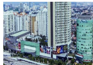
Tropicana City Mall & Tropicana City Office Tower, Petaling Jaya
