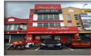
(C) Outlets at shophouses
